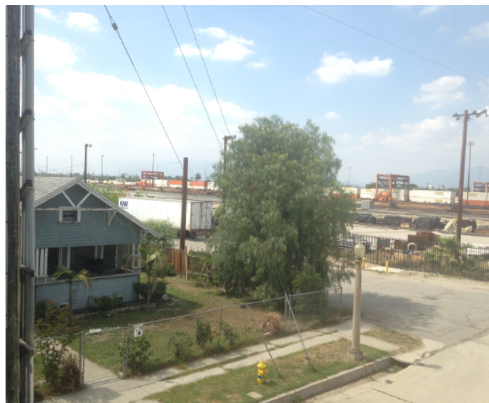
Homes next to the BNSF Railyard in Westside San Bernardino with the highest cancer risk of all railyards in the state.
